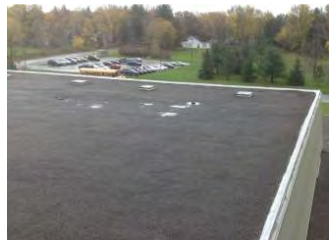
New Roof/ Restoration
